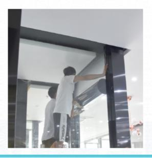
**Step 2.6:** Pull away the protective layer slowly and allow the FILM to adhere to the glass under its own weight. Starting at the top, use the roller in a horizontal (side-to-side) motion, gradually moving down the glass to disperse any air bubbles. If air bubbles still persist, carefully lift the FILM, check if any dust particles have stuck to the adhesive side and remove them with adhesive tape if so, and let the FILM settle again without air bubbles. See photos below.
